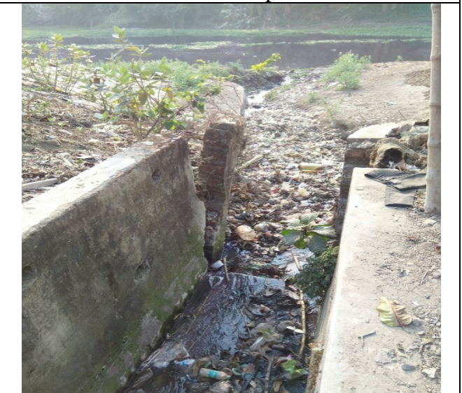
Drain at Barabazar ferry ghat
