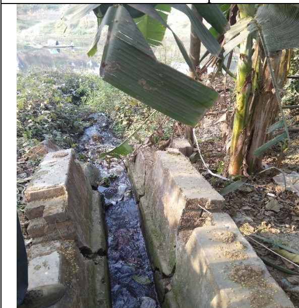
Drain at Samshan Ghat
