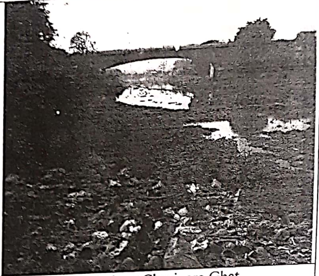
Drain at Churipara Ghat
