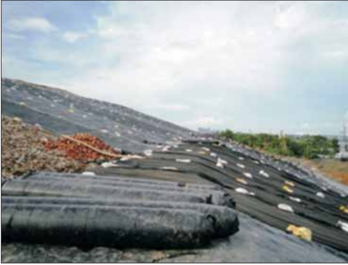
Laying of HDPE Cover
