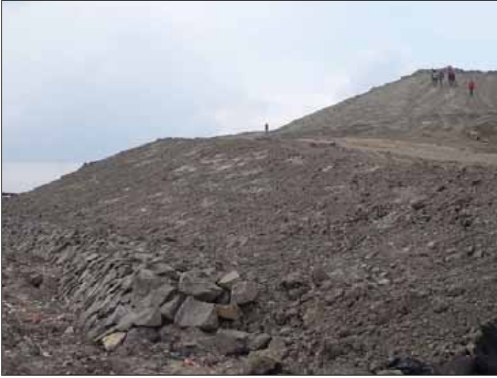
Laying of soil
