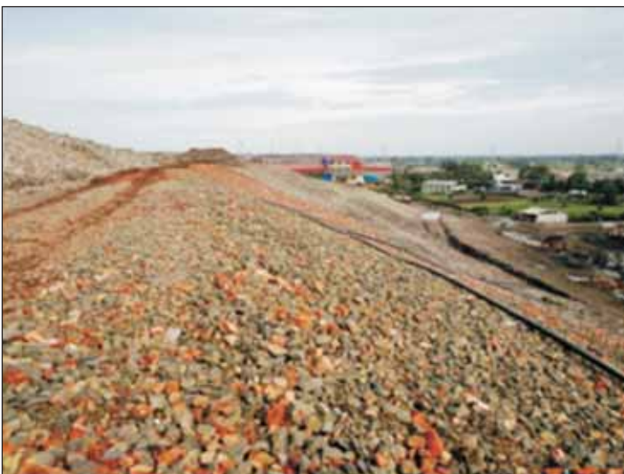
Gas drainage Layer
