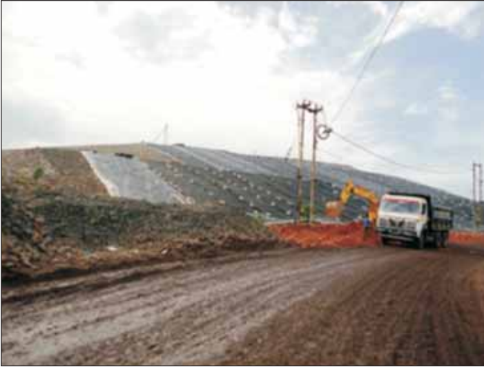
Laying of HPPE Cover
