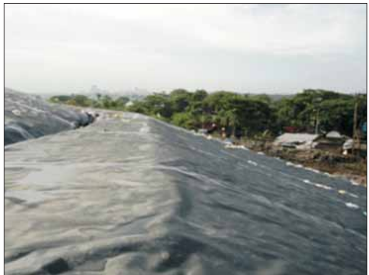
HDPE cover over berm
