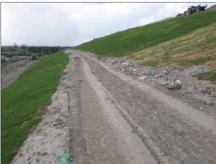
View of levelled surface
