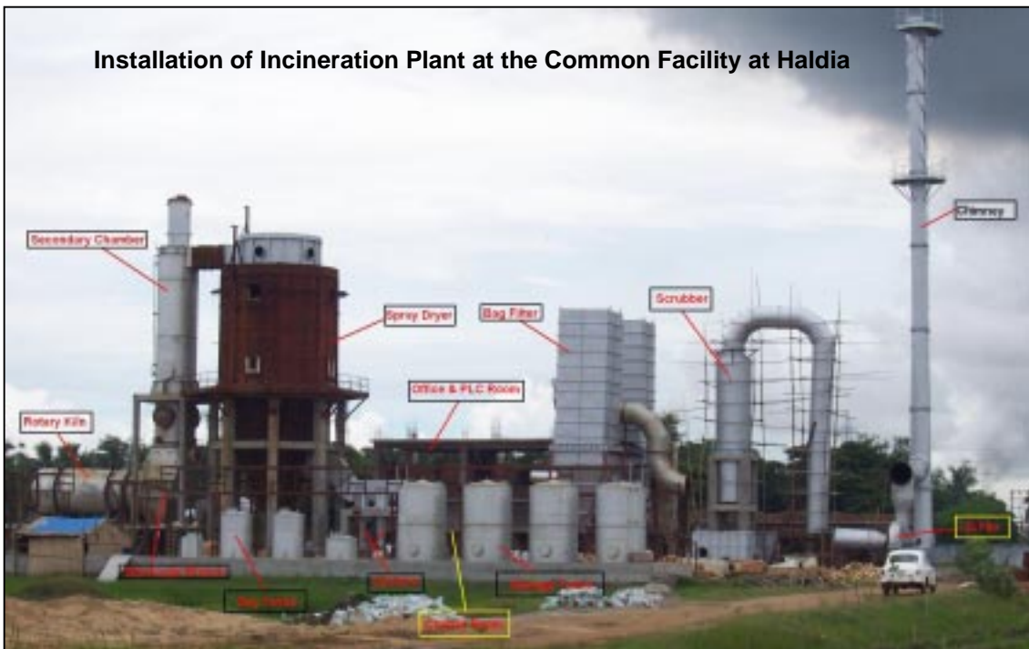
Installation of incineration plant at the common facility at Haldia
