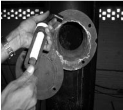
Stack Monitoring for PM
