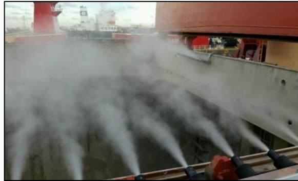
DRY FOG DUST SUPPRESSION SYSTEM
