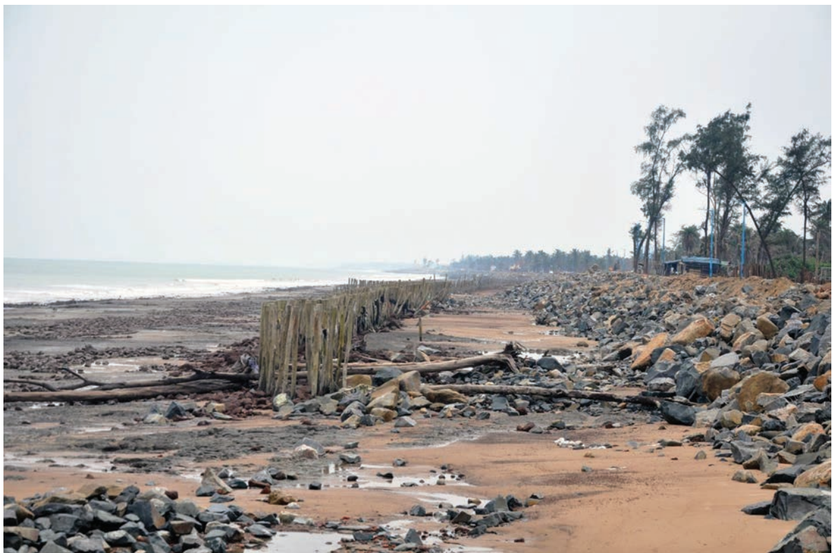
Fig. 41 Engineering intervention with boulders could not resist the encroaching sea
