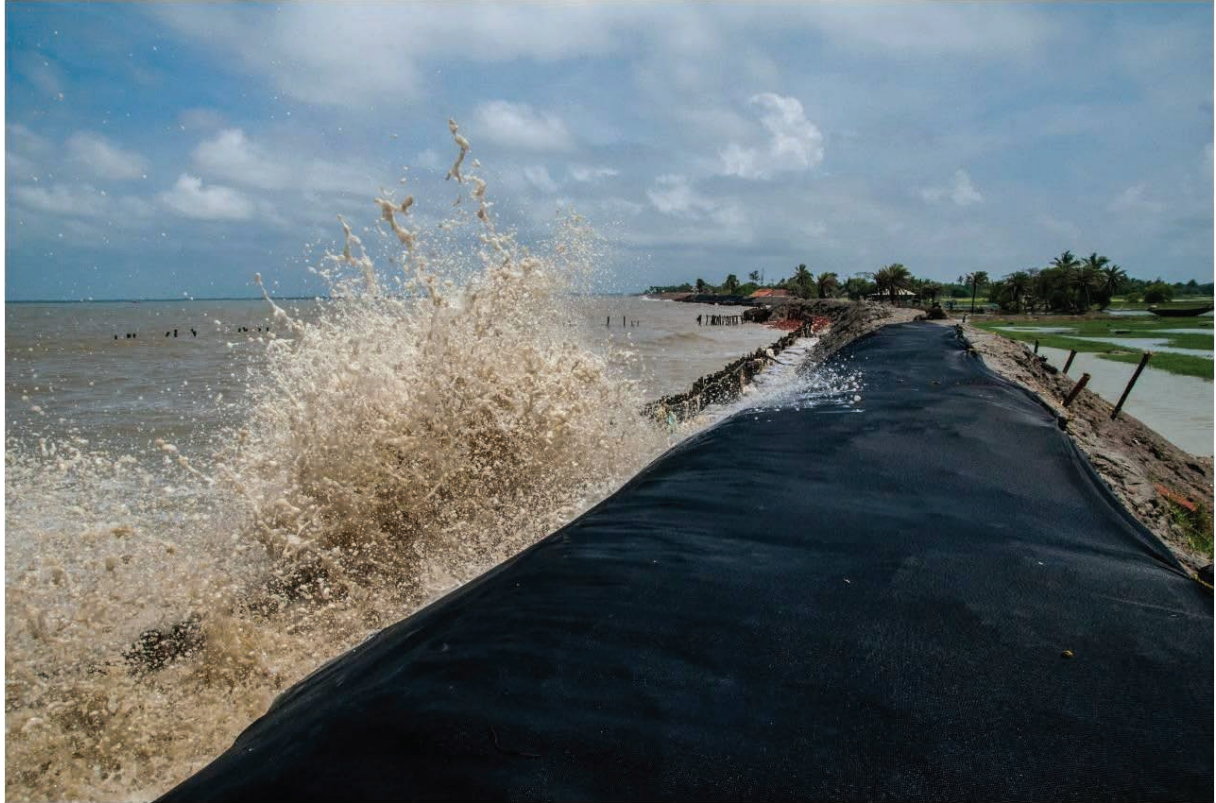
Fig. 5 Overtopping of coastal embankment
