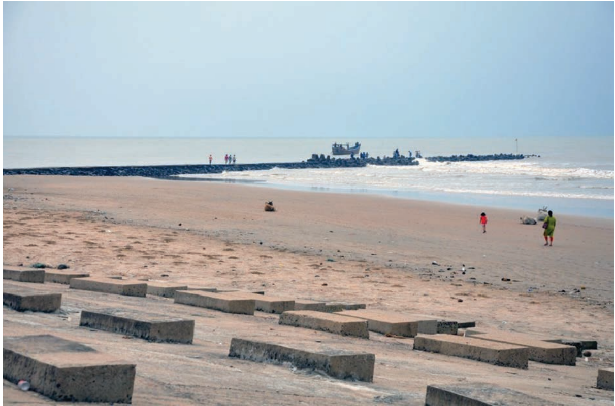
Fig. 40 The groyen built in 2009-10 has intercepted off-shore drift of sediment and created new beach
