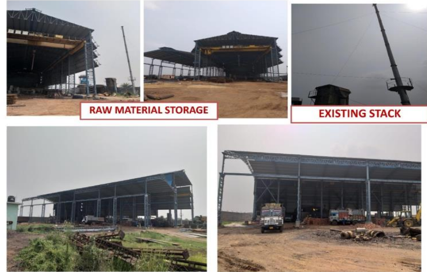
PHOTOGRAPH SHOWING THE EXISTING PLANT
