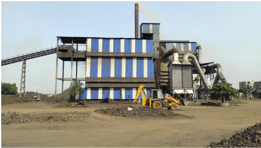
Figure-1.1 PHOTOGRAPHS OF THE EXISTING PLANT
