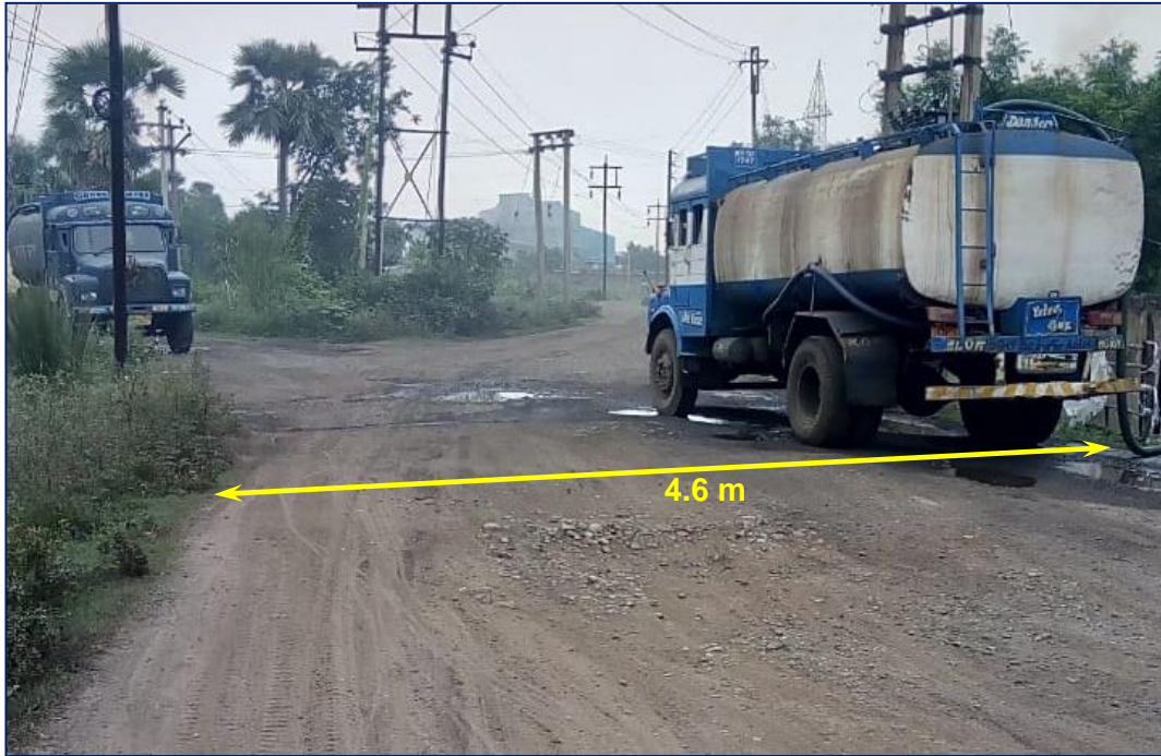
FIGURE-1.8 Panchayet Road adjacent to Project
