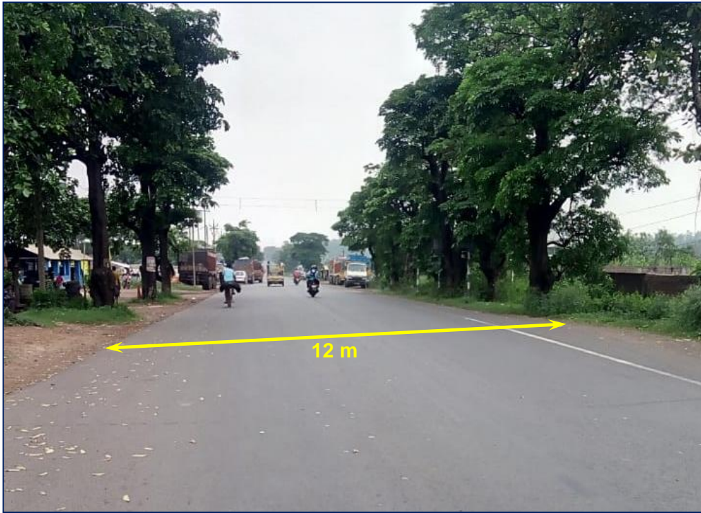
FIGURE-1.6 Durgapur-Bankura connecting State Highway - 9
