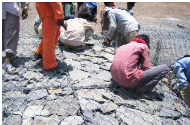
Figure 2.10: Lid closing operation
