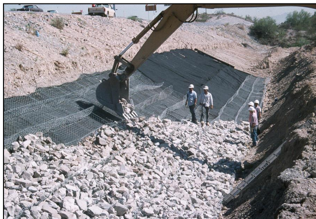
Figure 2.9: Filling of rocks in mattress units
