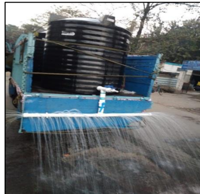
Water sprinkling on roads
