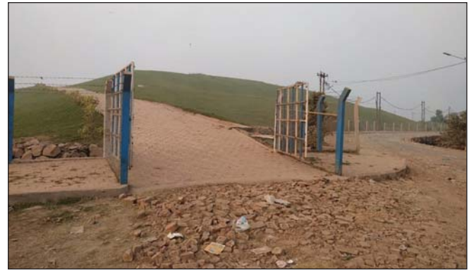
Figure 24.25: Construction of Service Road Over the Closed Dump Site
