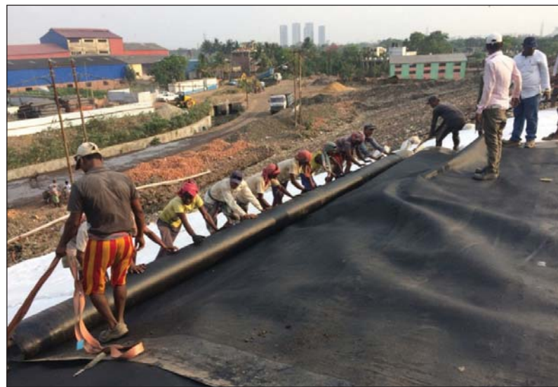
Figure 24.16: Installation of 1.5 mm thick HDPE Liner
