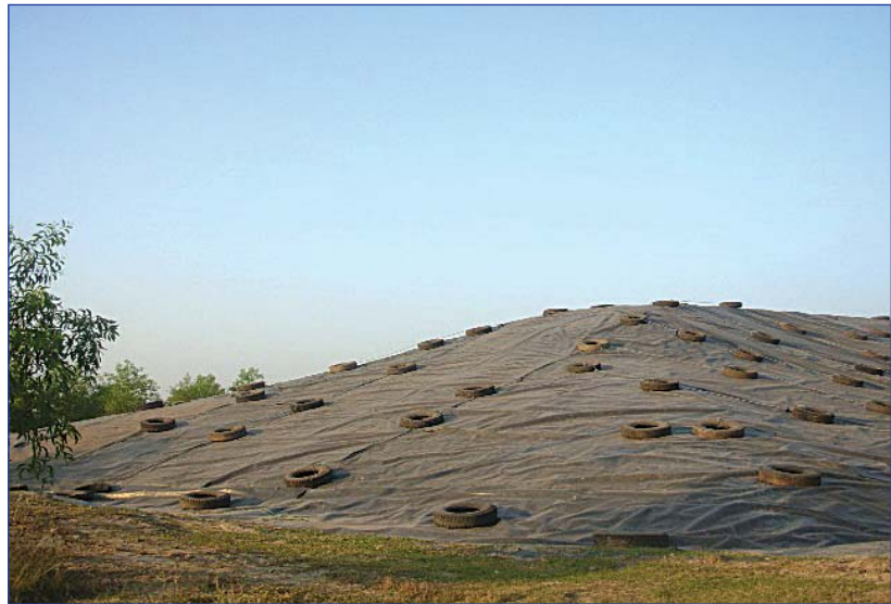
Phase -1 under Capping
