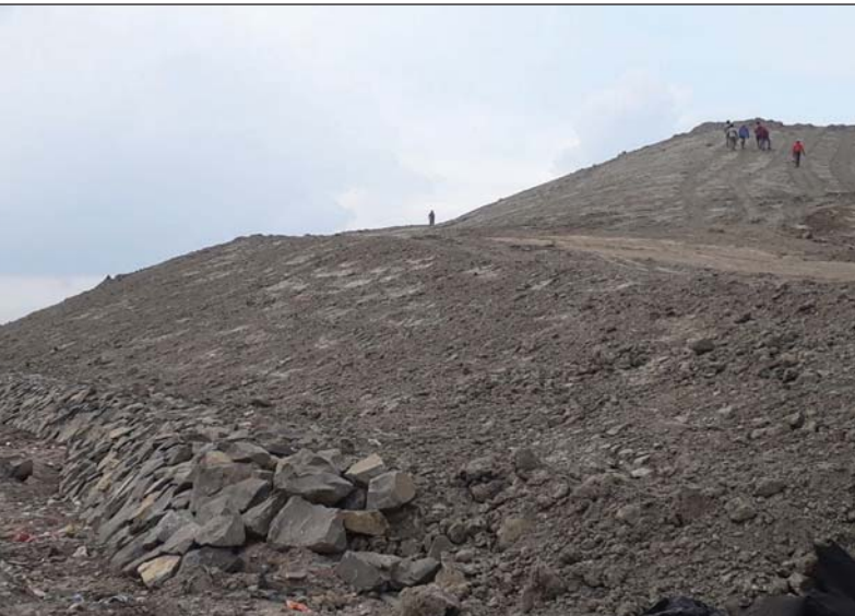
Figure 24.21: Laying of Clean Vegetative Soil
