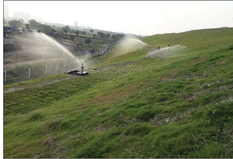
Figure 24.28: Installation of Irrigation System
