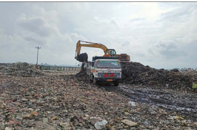
Figure 18(I).7: BMC Dumping Site, Mollar Bheri -Preparation of Bio-mining is going on
