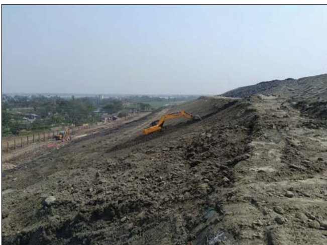
Figure 24.18: Laying of 500 mm thick non-contaminated soil layer
