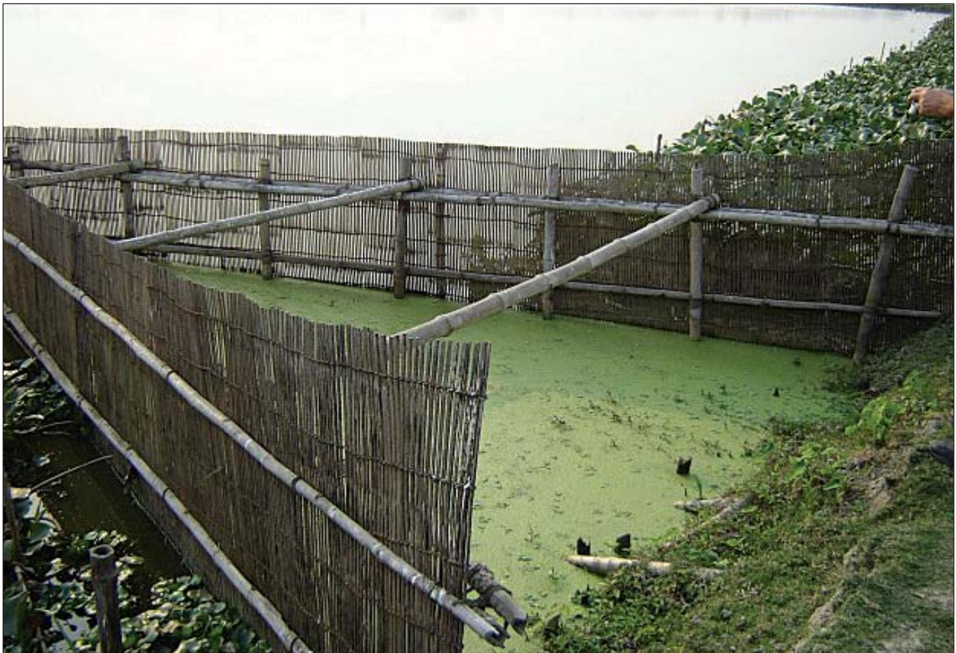
Figure 12.9: Bamboo screens used for filtering solids from sewage before entry into ponds
