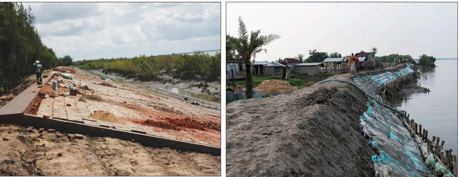
Figure 13.7: Earthen Embankment and Concrete Embankment.
