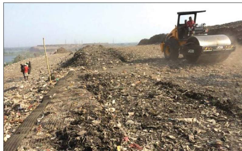
Figure 24.20: Installation of Geo Reinforcement Mats
