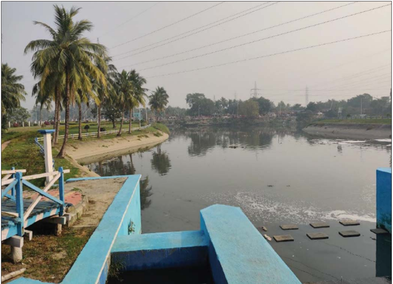
Figure 12.3: Bantala Lockgate, where the sewage enters EKW
