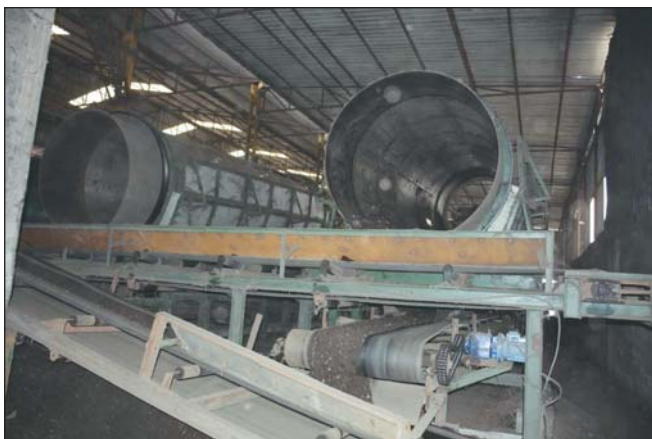
Figure 18(I).3: Trommel Installed for Bio-mining at Dhapa
