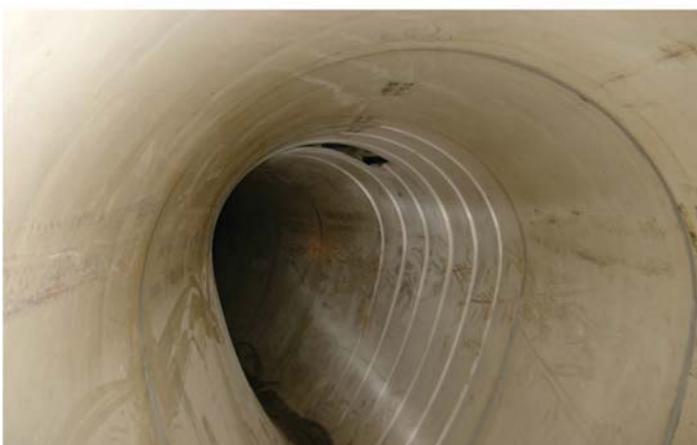
Figure 19.12: The top left image shows the narrowing of the drainage pipes due to siltation. The right image shows the process of retrofitting done on the existing brick sewer using trenchless technology. The bottom left image shows the completed section of GRP liners.
