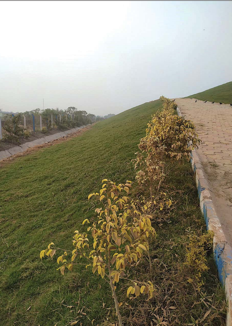
Figure 24.27: Laying and Planting of Hedge/Shrub
