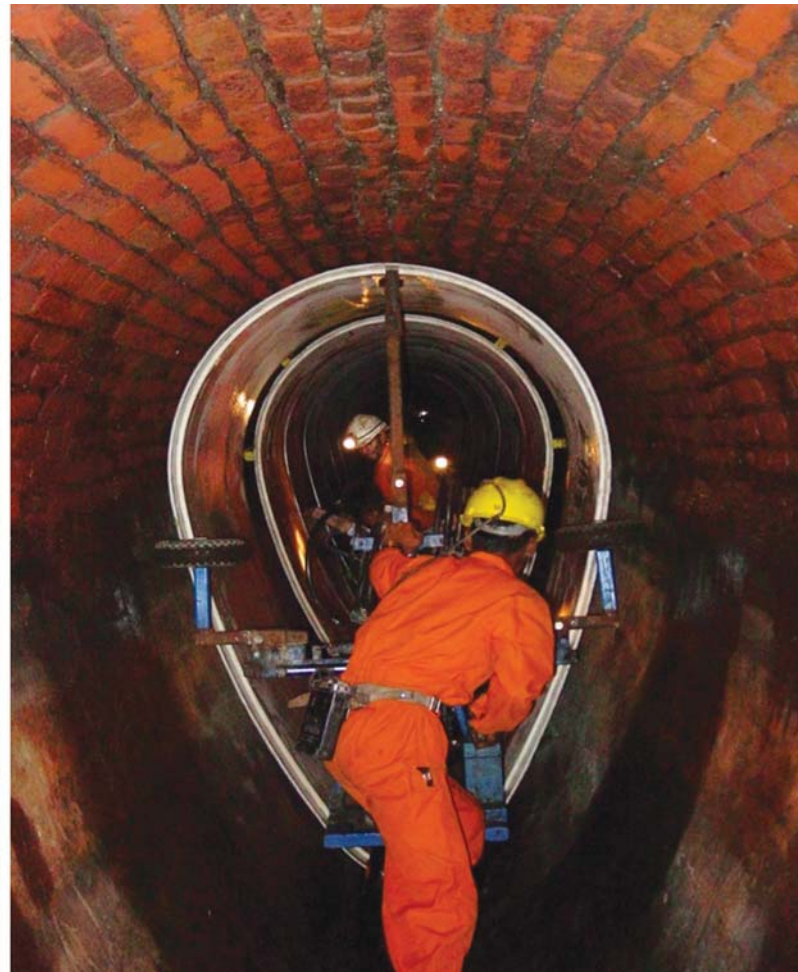
Figure 19.12: The top left image shows the narrowing of the drainage pipes due to siltation. The right image shows the process of retrofitting done on the existing brick sewer using trenchless technology. The bottom left image shows the completed section of GRP liners.
