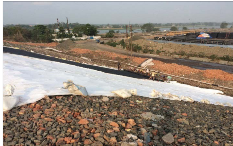
Figure 24.15: Installation of Non-woven Geo Textile
