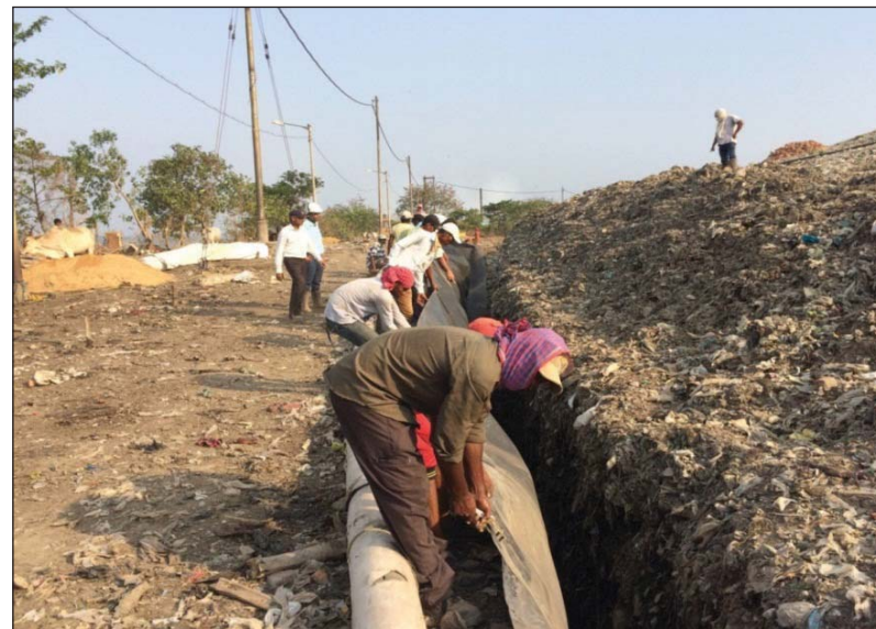
Figure 24.12: Construction of Peripheral Leachate Collection System
