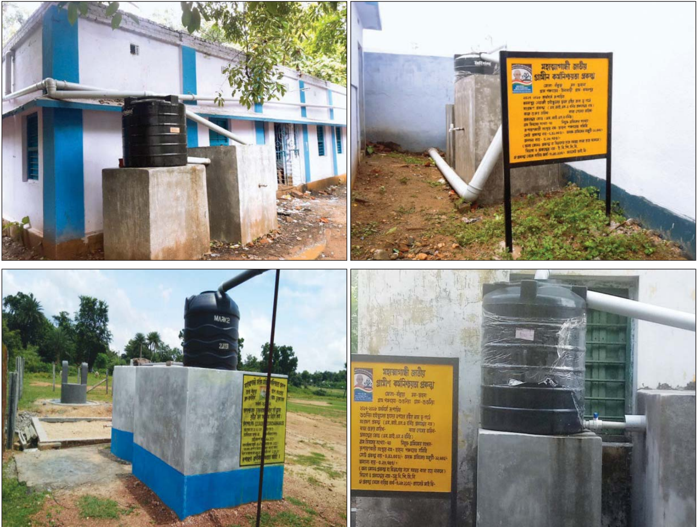
Figure 24.10: Rainwater Harvesting Structures
