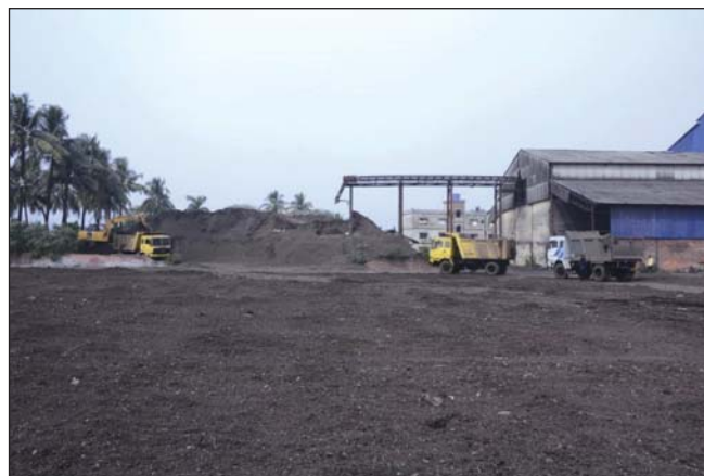
Figure 18(I).4: Compost Plant at Dhapa
