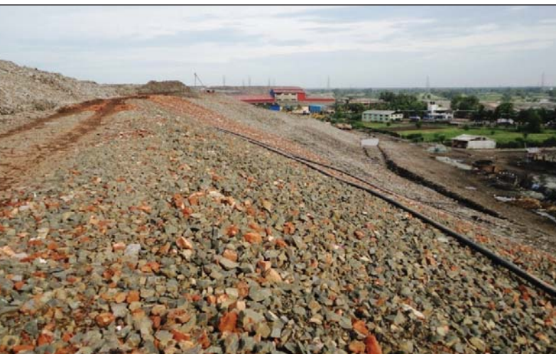
Figure 24.14: Gas Drainage Layer
