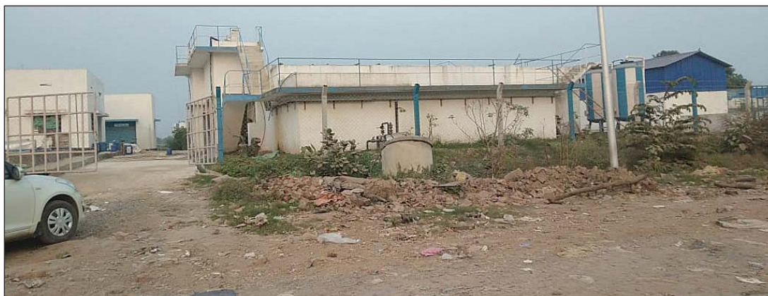
Figure 24.30: Leachate Treatment Plant
