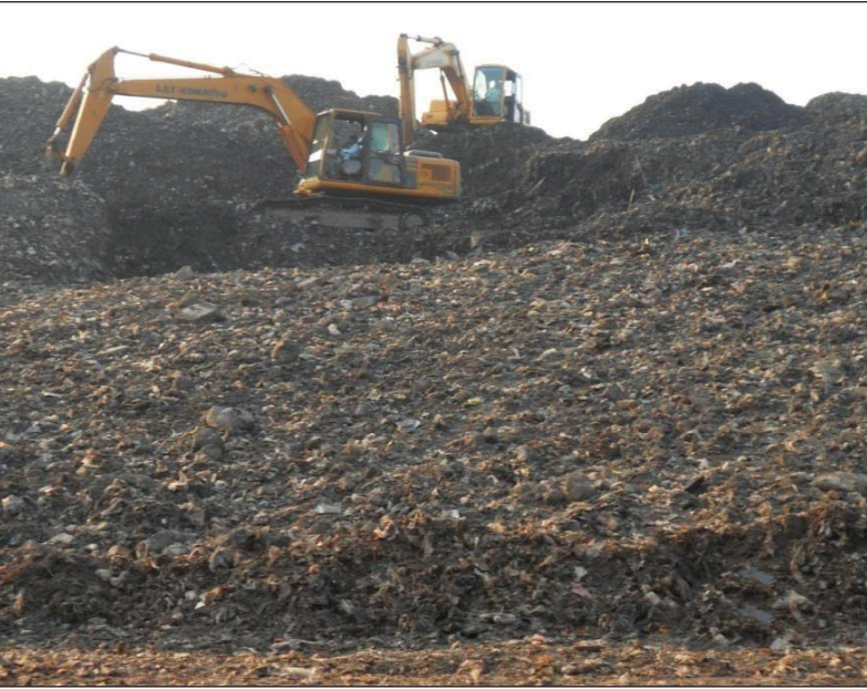
Figure 24.13: Profiling & Reshaping of Dumpsite
