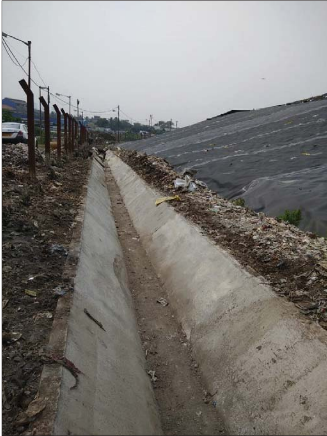
Figure 24.24: Construction of Storm Water (Surface Water) Drainage System
