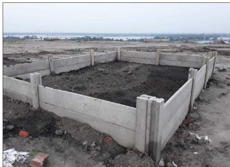
Figure 24.23: Construction of Compost Filter Boxes: 10 nos.
