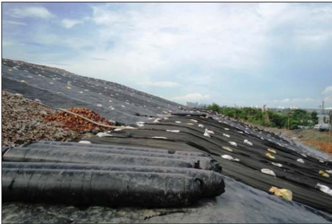
Figure 24.17: Installation of Geo Composite (Drainage Mat)
