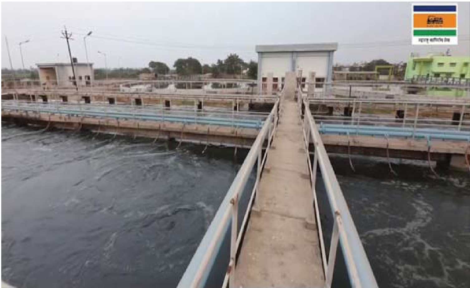
Figure 19.11: The Largest Wastewater Treatment Plant in Nashik
