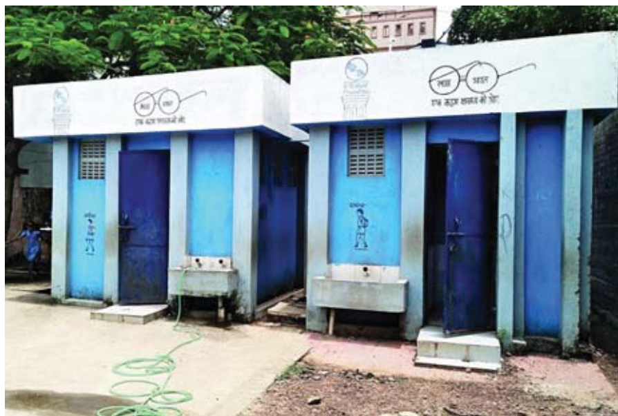
Figure 19.14: Construction of Toilet Facilities under the Swachh Bharat Mission
