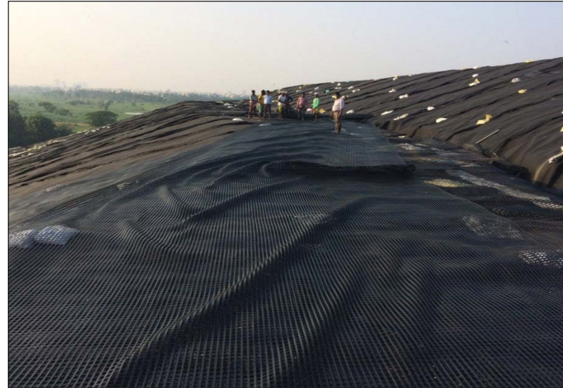
Figure 24.19: Installation of Geo Reinforcement Grid
