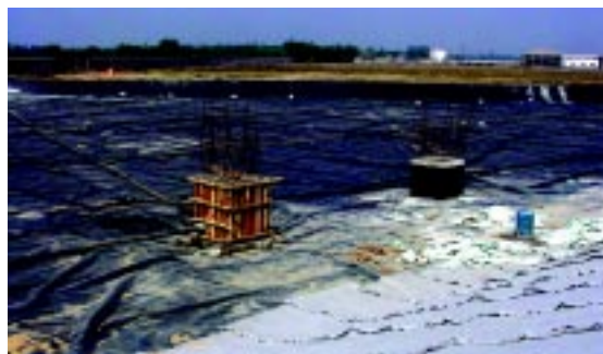
First Cell of the Landfill facility of Common Treatment, Storage and Disposal Facility for hazardous waste at Haldia 1
